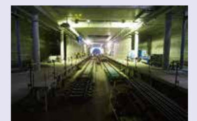
View of preparations for route heading to eastern part of Kanagawa
