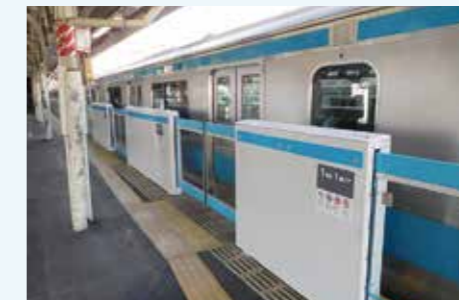
Example of platform doors (Tsurumi Station's JR Keihin-Tokaido Line)
