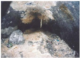
Sewer pipe blocked with oil
