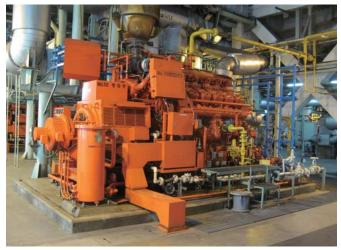
Gas generator for electricity generation running on digestion gas
