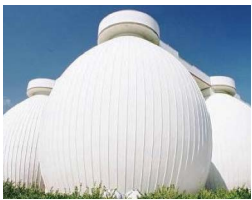
Egg-shaped digestion tank
