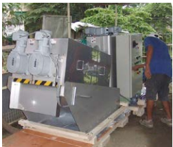
Sludge dewatering equipment installed
