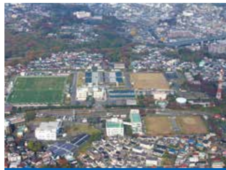
Nishiya Purification Plant
