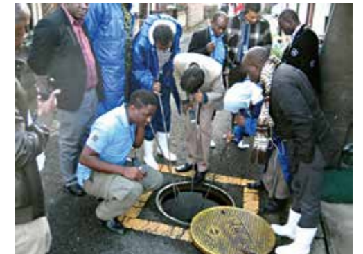
Training for leakage detection with acoustic rods
