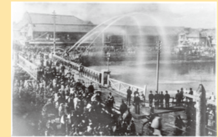
A sprinkler at the time of foundation
