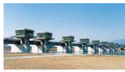
Sagami ohzeki intake weir
