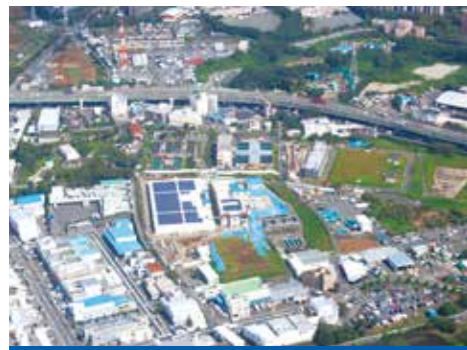
Kawai Purification Plant
