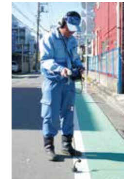
Leakage detection work
