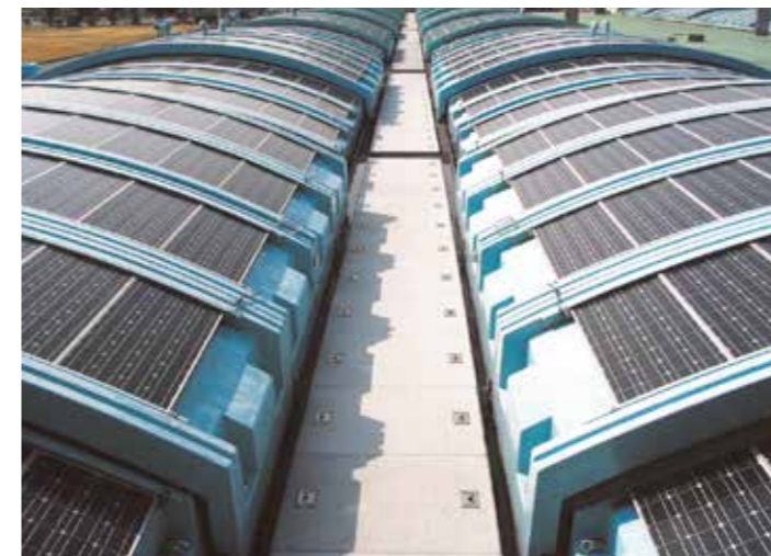
A movable solar power generation system above a filtration basin (Kosuzume Purification Plant)
