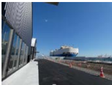
Continuous berth that extends over 1,000m.
