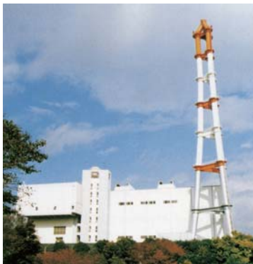
改修前施設外観 Facilities before renovation
