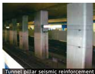
Tunnel pillar seismic reinforcement
