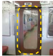
● Gangway door (prevent fire from spreading)
