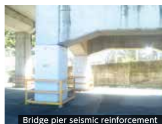
Bridge pier seismic reinforcement
