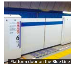
Platform door on the Blue Line
